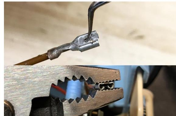
14. The picture at right shows how the spade terminals will properly lock together in later steps. Do not perform this step yet.
